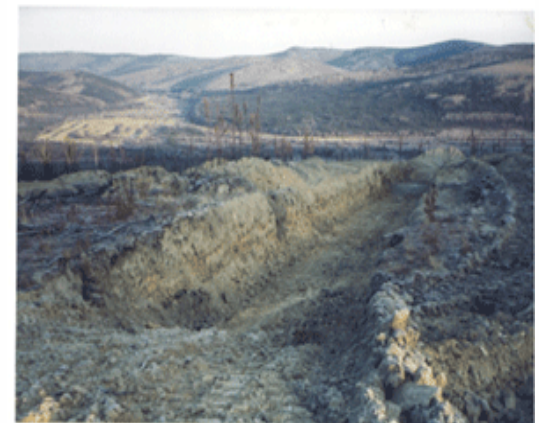
GIL EXTENSION - TRENCHING
