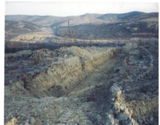
GIL EXTENSION - TRENCHING
