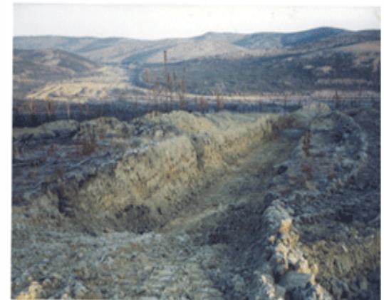
GIL EXTENSION - TRENCHING
