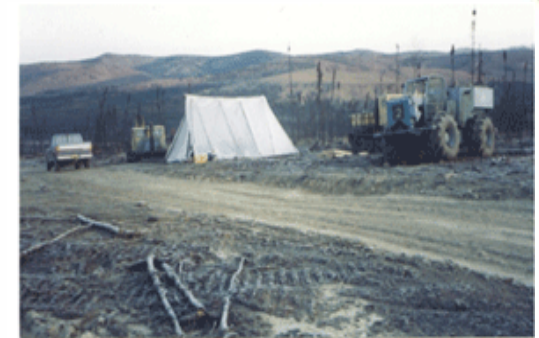
GIL EXTENSION - SUPPORT EQUIPMENT
