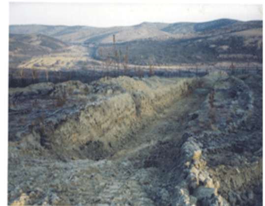
GIL EXTENSION - TRENCHING
